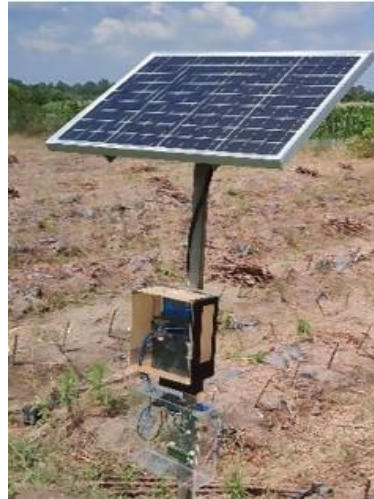
Figure 2. overall solar PV
